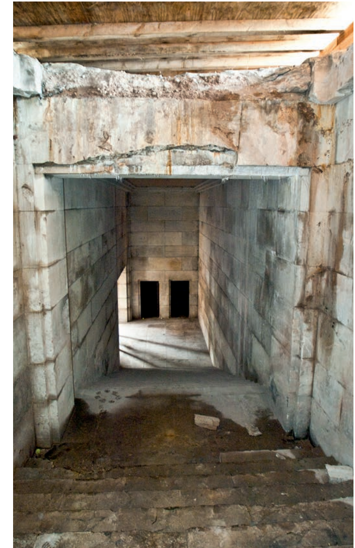
A cleared stairwell inside the Zeppelin Grandstand.
