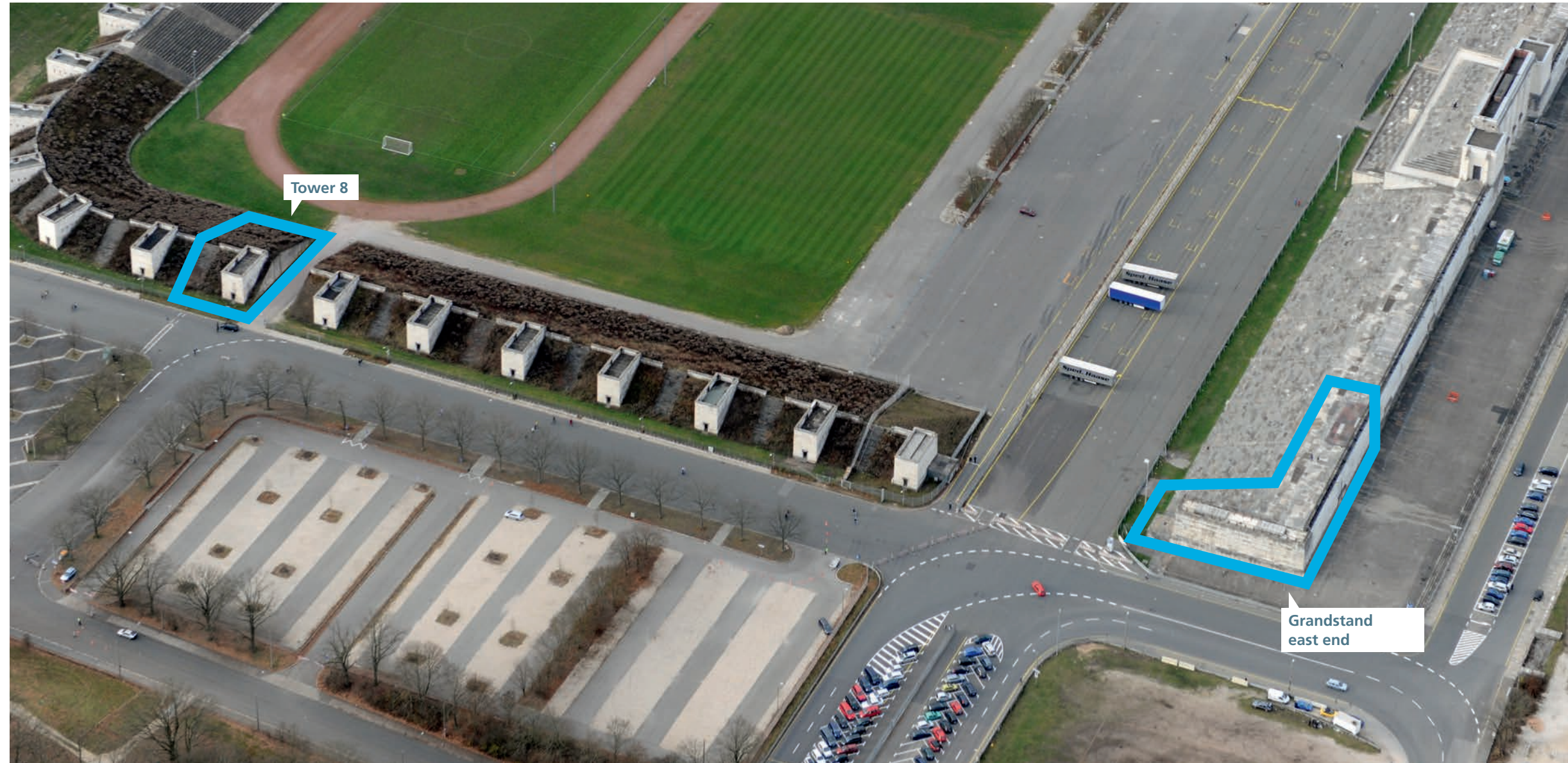
The marked sample areas were be thoroughly investigated in autumn 2013. Based on the results, they will be refurbished in 2015.
