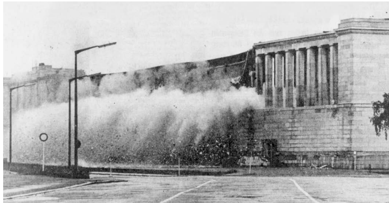
Demolition of the rows of pillars on the Grandstand, 1967.
