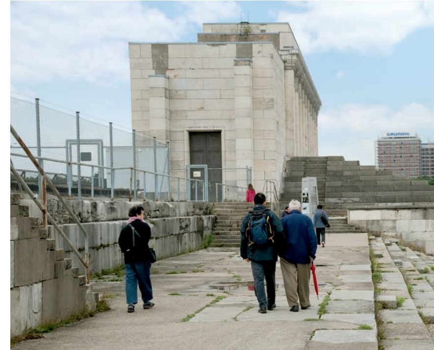
Visitors next to fenced-off areas (left) on the Zeppelin Grandstand.
