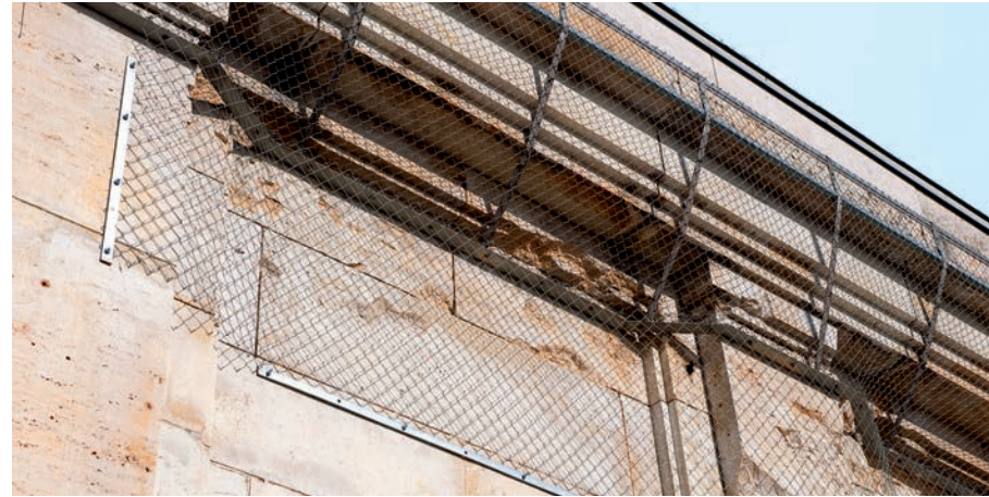
Securing crumbling ledges with wire mesh.
